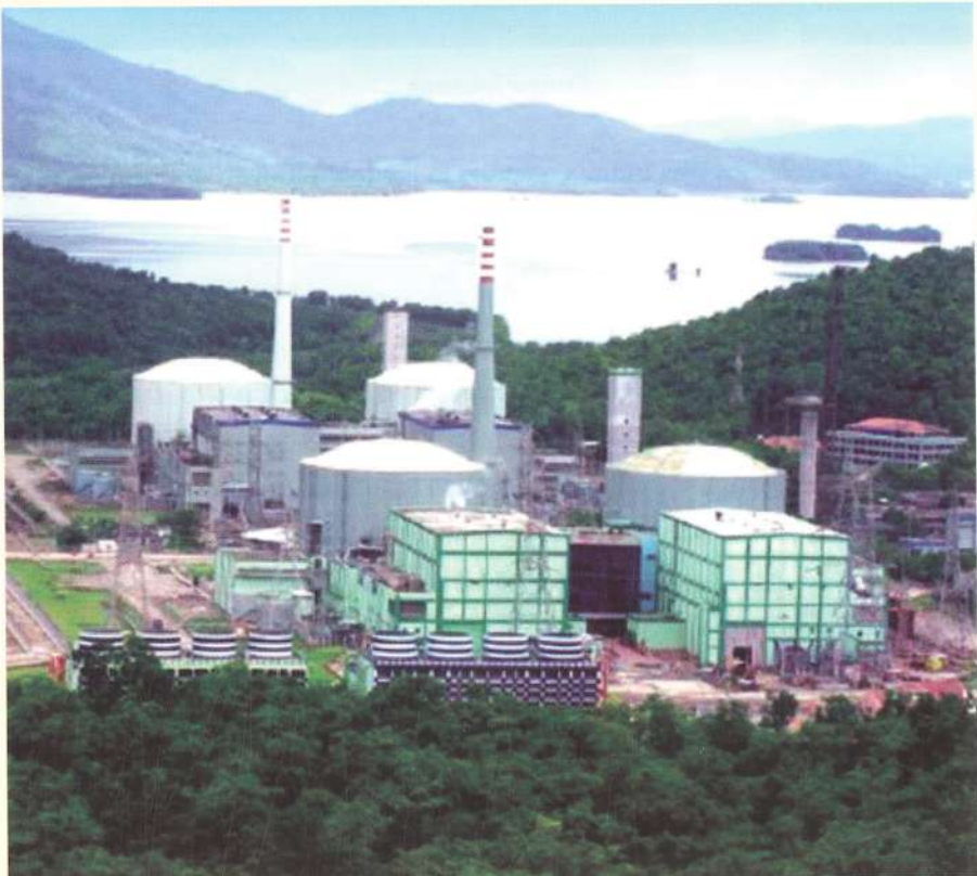
Fig. 2.11 Kaiga Atomic Power Station (Four Units).
