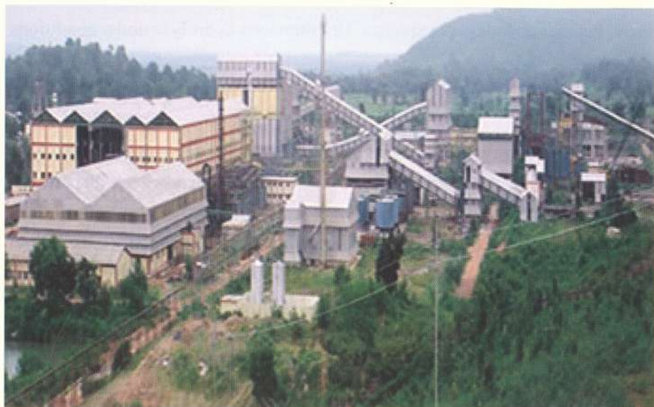
Fig. 3.6 A view of the Turamdih Uranium Mill.
