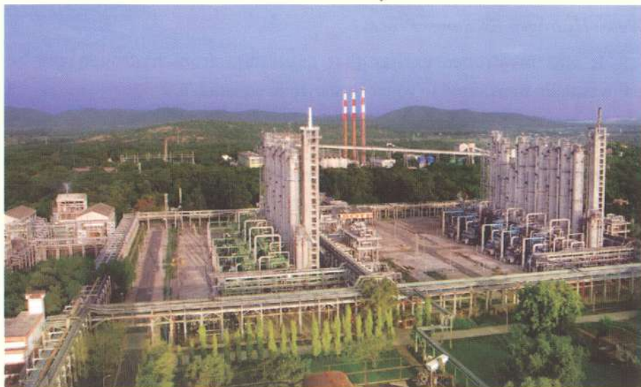
Fig. 6.4 A view of the Heavy Water Plant at Manuguru
